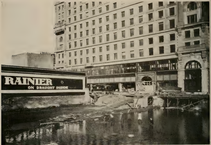
Market and Powell streets, San Francisco, on February 1, 1907, nearly one year after the big conflagration. The excavation in the foreground, flooded by the winter's rain, is where the massive concrete foundations of our majestic home were laid thirteen years later.
